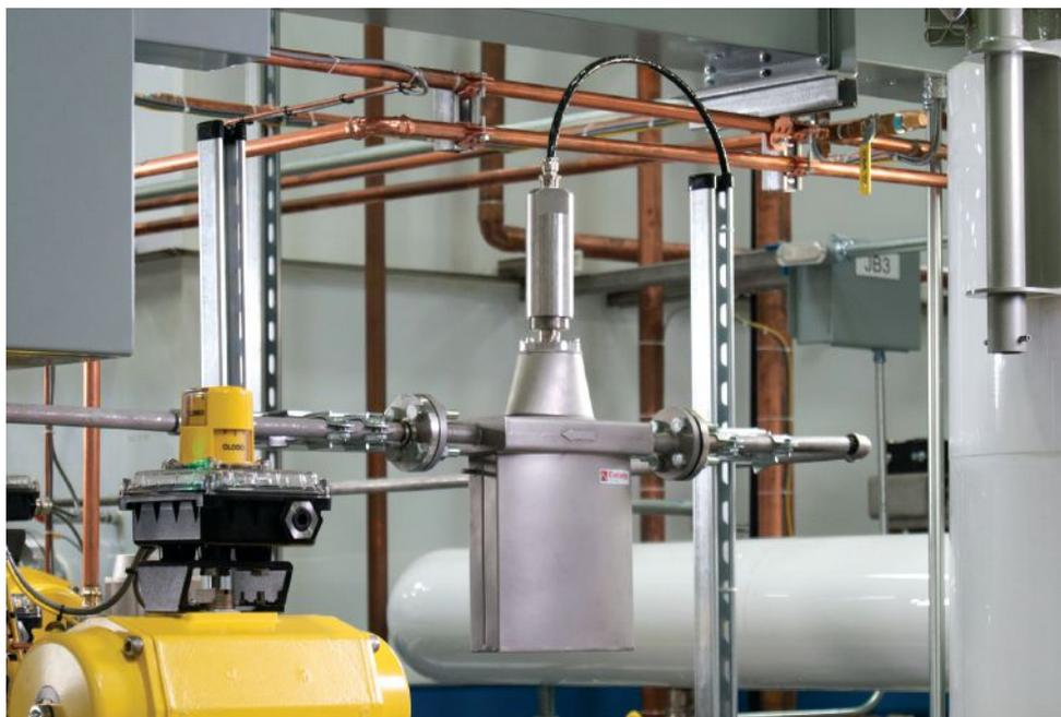
Image 1. Coriolis flow meters are designed to directly measure fluid mass over a wide range of temperatures with very high accuracy. (Images courtesy of Badger Meter)
