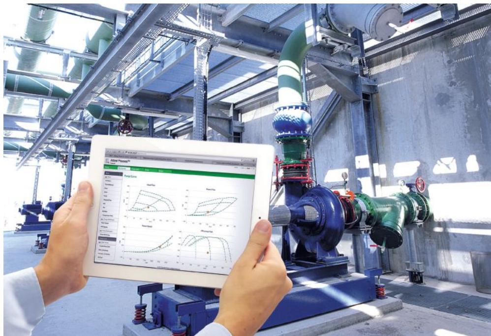
Image 1. Tracking pump output levels through a browser-based monitoring application for variable frequency drives using a handheld device (Image and graphics courtesy of Schneider Electric)
