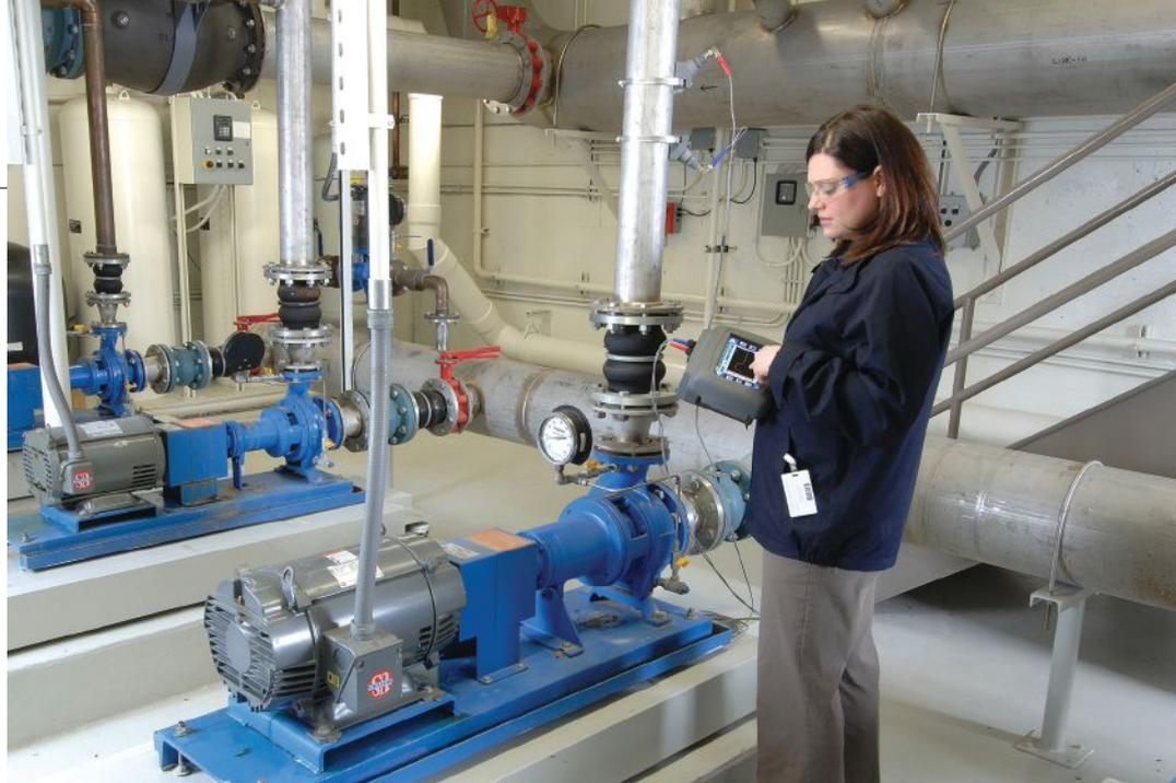
Image 2. Clamp-on ultrasonic flow meters can be used for troubleshooting a wide range of flow issues, from verifying the reading of another meter to monitoring flow systems over an extended time period.
